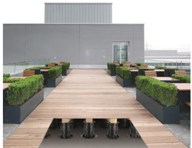
Fig. 6: EnBW, roof terrace, combination timber&stone, underconstruction PLV50/75 and ZSt65/100, 135-170 mm.
