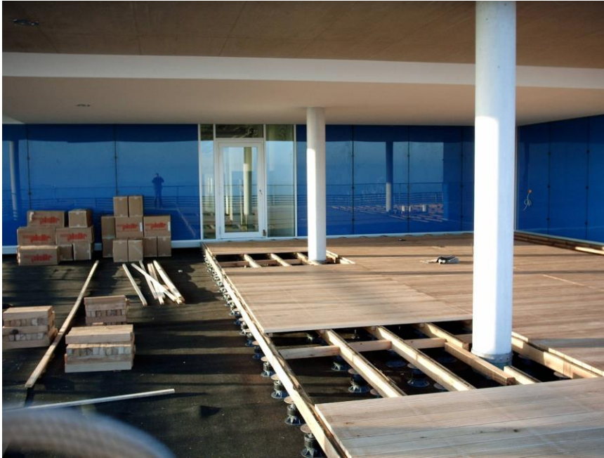
Fig. 3: Pedestals PP155/15, PP155/45 stacked, combined with height adjustable PLV50/75. Project MPI Tübingen.
